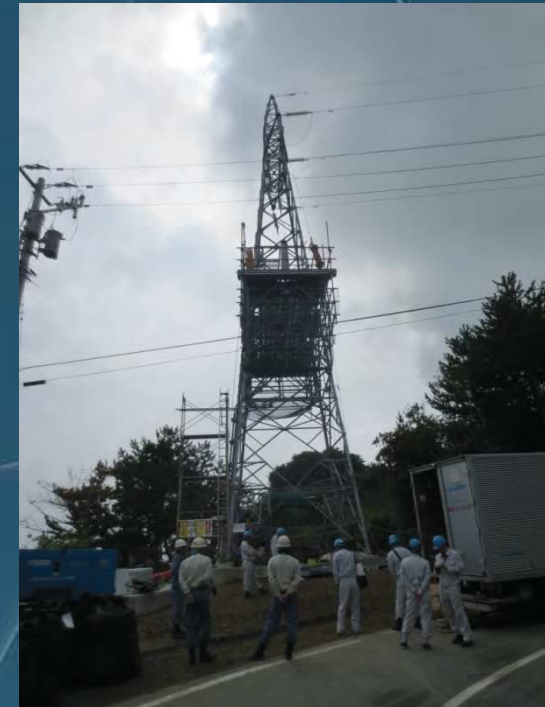
On-site test for 66kV Cable
