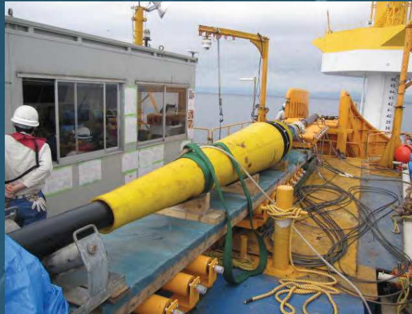
22kV riser laying at S/S
