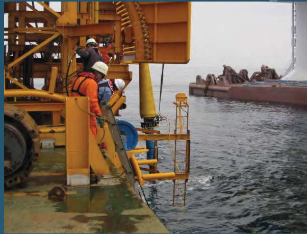
66kV riser laying at S/S
