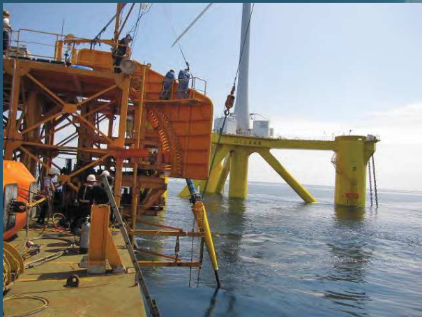
22kV riser laying at turbine
