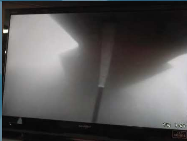
22kV riser below turbine
