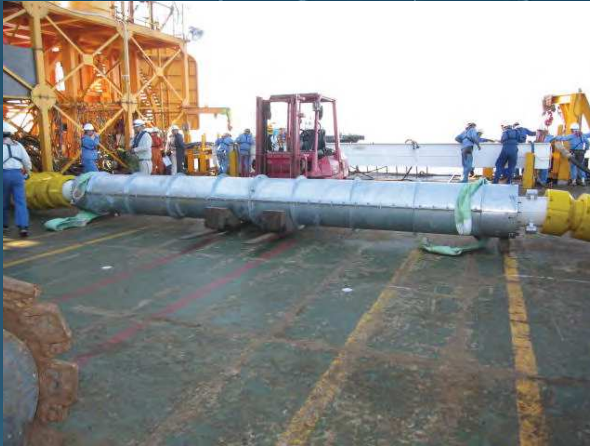
66kV transition joint on the laying vessel
