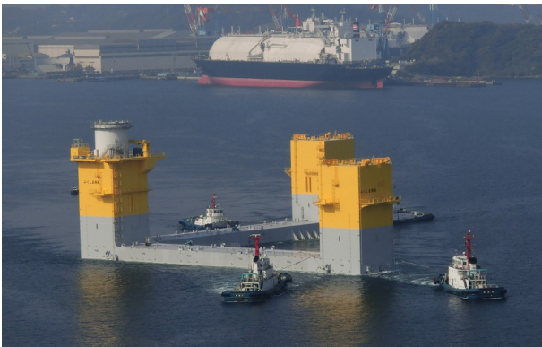
Fig.8 Floating Structure during Towing
