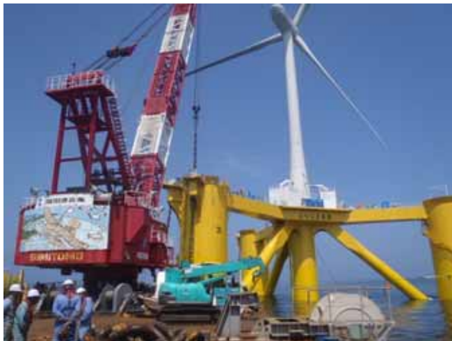
Connecting chain to the floater
