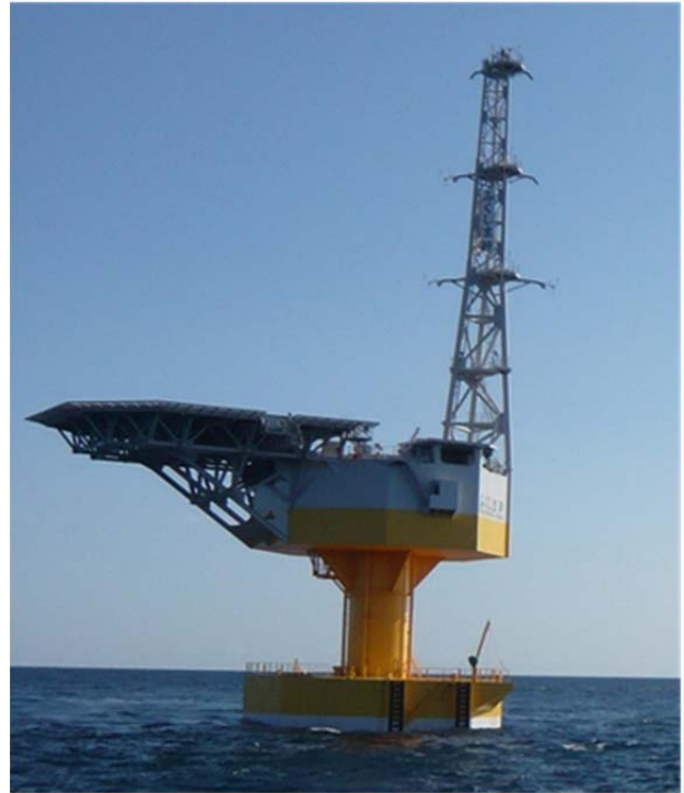
Fig. 9. Floating substation installed
