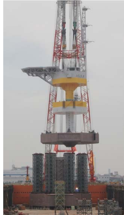
Fig. 5. Mega block installation on lower hull part.
