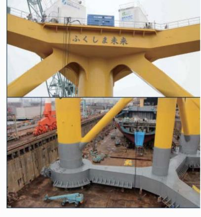
World first 2MW downwind offshore wind turbine was installed on the compact semi-sub floater in June, 2013. The 55m tower was divided into three sections and after the installation of the nacelle, 40m blades were installed.
