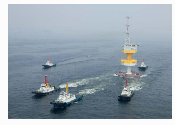
The advanced spar floater for floating substation left Isogo dock of JMU and towed to the installation site directly. From the 16th of June, 2013, the anchoring began.
