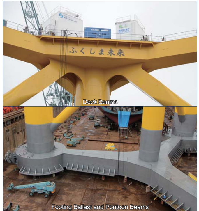
Footing Ballast and Pontoon Beams
