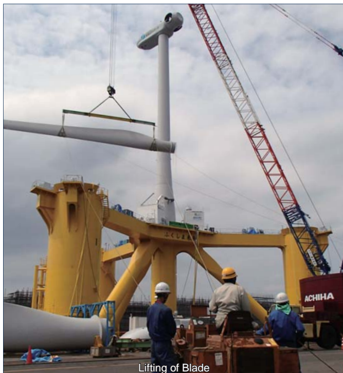
Lifting of Blade
