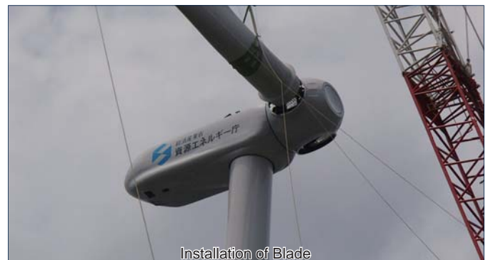
Installation of Blade
