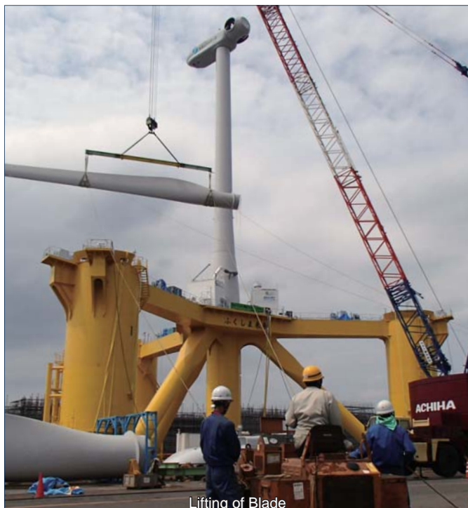
Lifting of Blade
