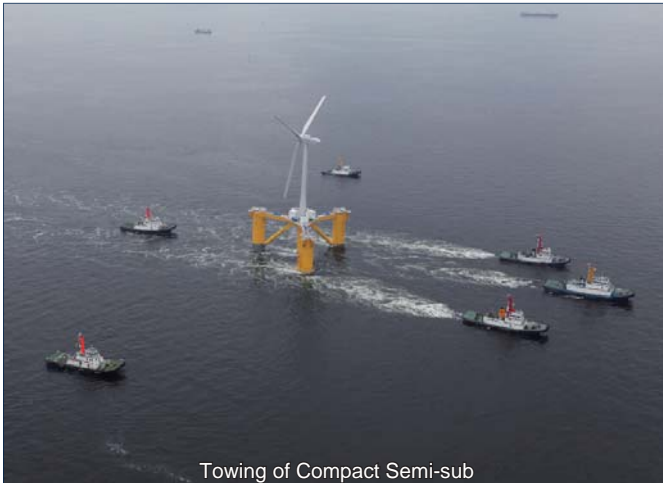
Towing of Compact Semi-sub
