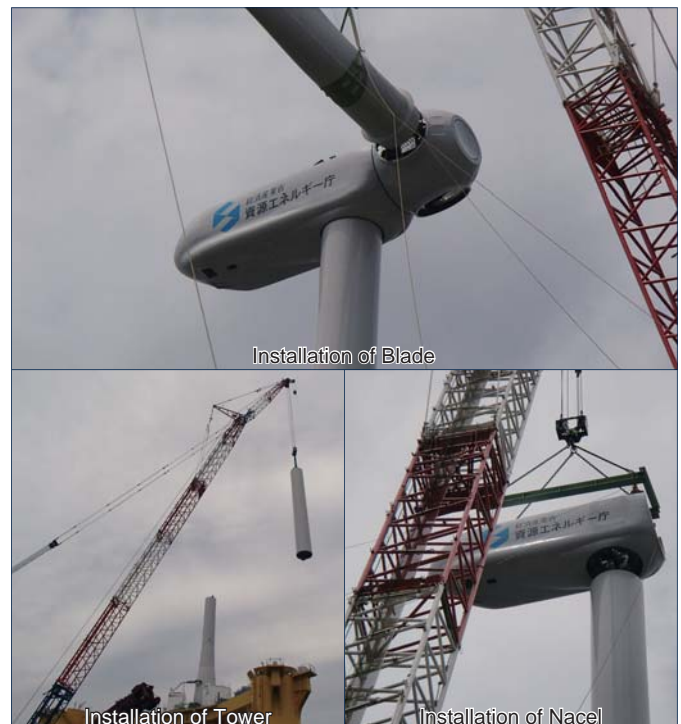
Installation of Tower
