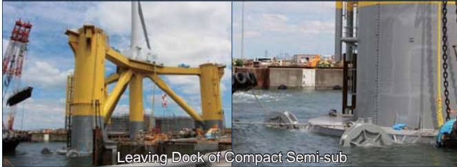
Towing of Compact Semi-sub
